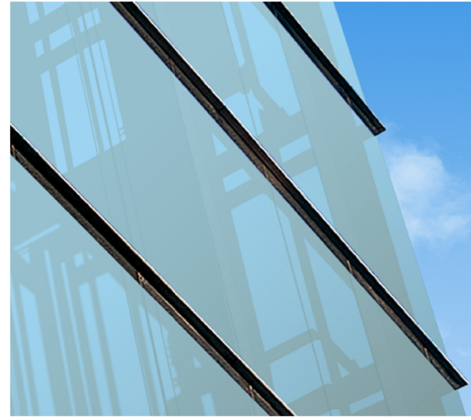
GLASS CURTAIN WALL - CLEAR SCREEN GL1
